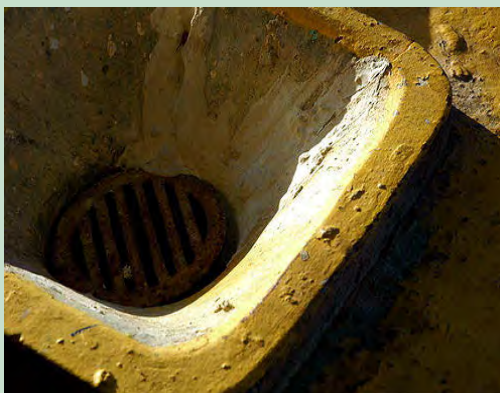
Drains and pipes.
