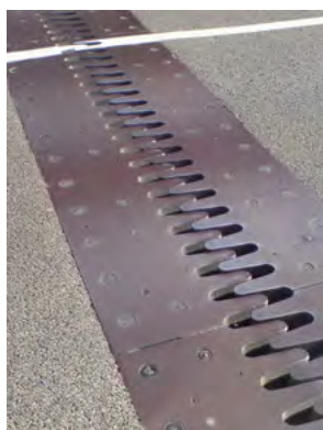
The expansion joint in a bridge.
