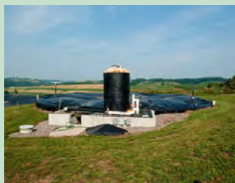
Biofuel- manure decomposes to produce methane gas.
